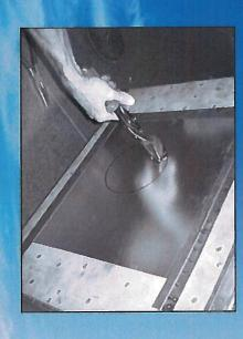
Cutters can now use the hole to begin cutting out the 6" outflow into the cold air return of the furnace
