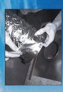
Use steel tape to seal the flex to the collar airtight.
