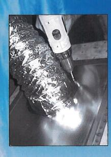
4 screws are needed to completely secure the collar to the return
