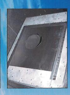
A 6" hole should now be cut into the cold air return right before it enters the furnace
