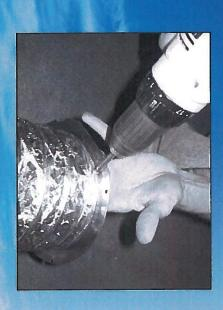
Secure flex to the duct with self tapping metal screws
