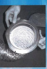
3 screws evenly spaced will secure the flex to the collar
