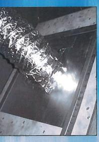
Steel tape around the 6" collar to make the connection to the cold air return airtight
